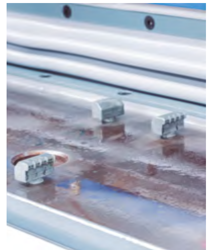
Figure 3.16. Blowers located on the perimeter of the bottom plate.
