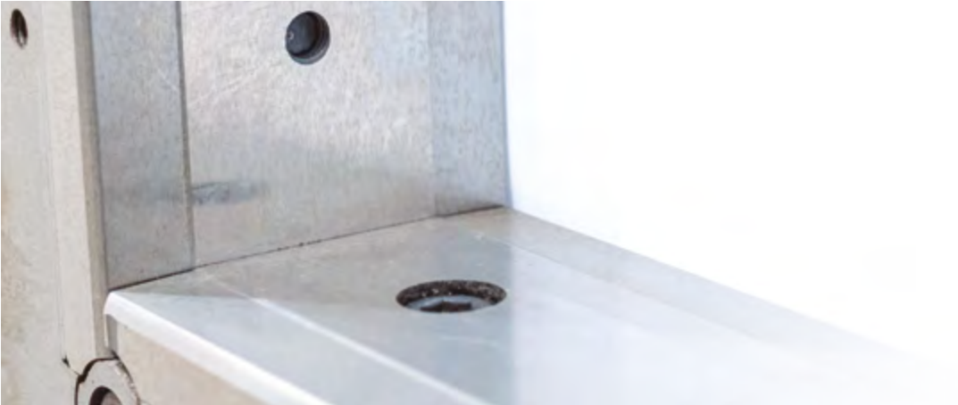
Figure 3.27. Reversible symmetrical liners (detail).
