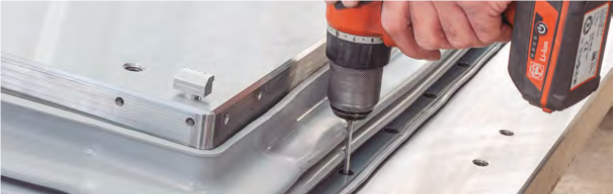
Figure 4.13. Assembly of bellows.
