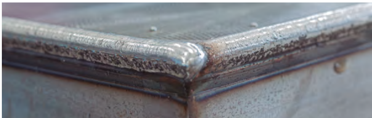
Figure 4.36. Perimeter weld bead.
